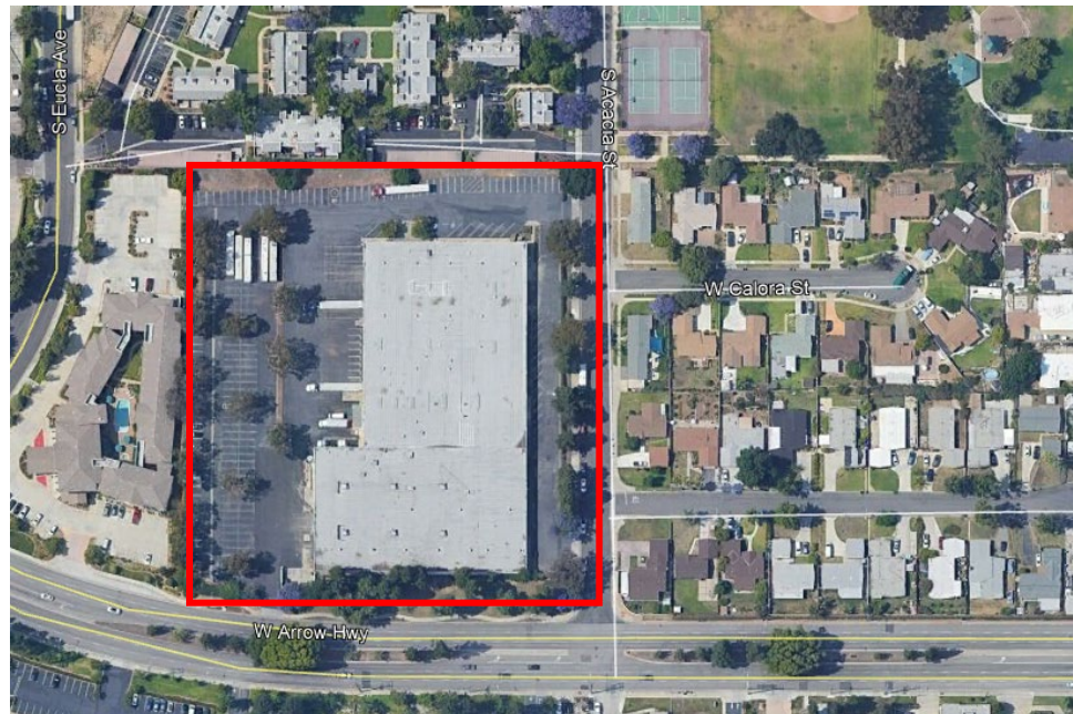
Figure A-8 Warehouse Site
